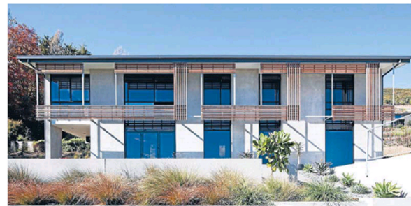
Tiltpanel house, Nelson 2009
